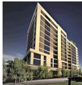
716 Main Street East (under construction)
