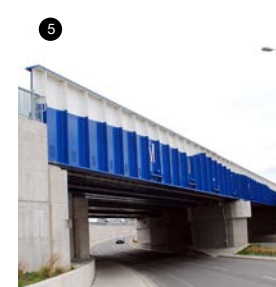
Rail bridge over Main St. E.
